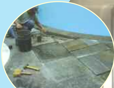
Pool Deck Renovation
