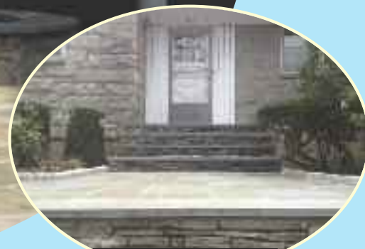
Retaining Wall & Steps
