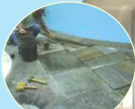
Pool Deck Renovation
