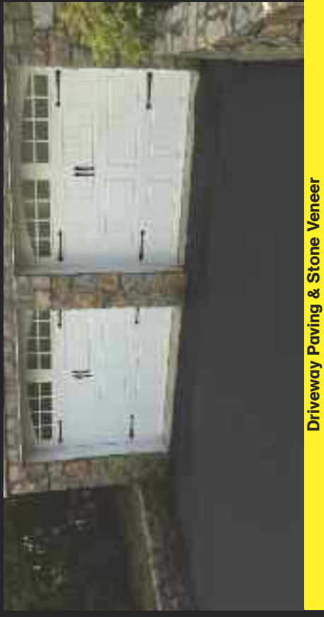
Blacktop Driveway w/Belgian Block Apron & Curbing
